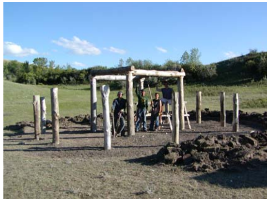
Construction of Mandan Earth Lodge Photo by Travis Hallam
