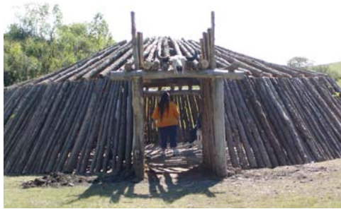
Construction of Mandan Earth Lodge Photo by Travis Hallam
